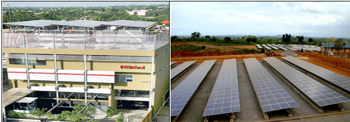
Figure 1. A solar roof (25 kW) on a commercial building in Colombo and one of the two solar farms (500 kW each) installed in Sri Lanka for initial training and promotional purposes.
